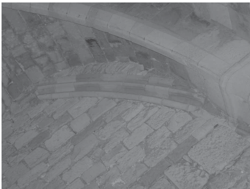
Fig. 24: Limassol Castle, réduit , detail of southern half of Gothic chapel transverse arch, now immured in later wall [M. Olympios].
